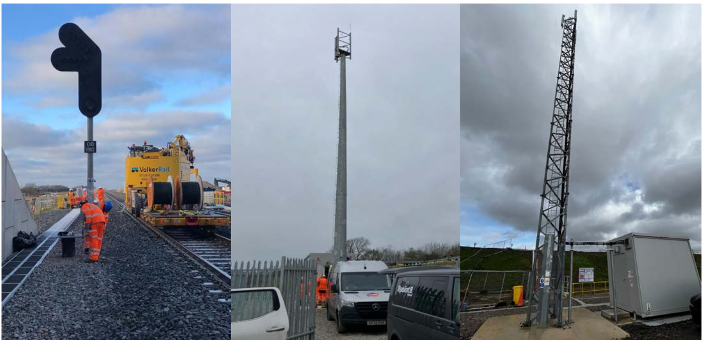
L-R: A signal installed on site, a tower and a lattice tower Global System for Mobile Communications-Railway mast.
