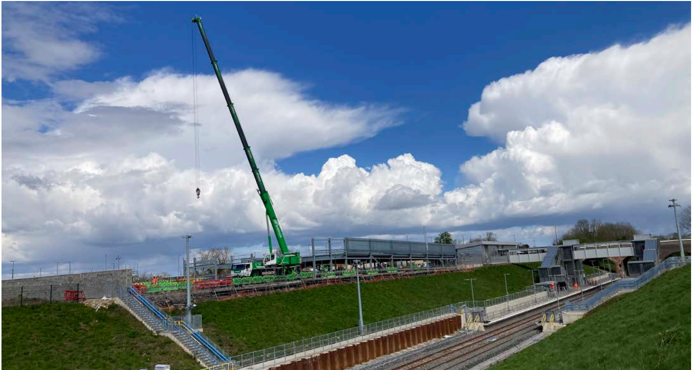
Winslow Station car park construction for Buckinghamshire Council in progress with a crane being used to lift the steel beams and place concrete panels
